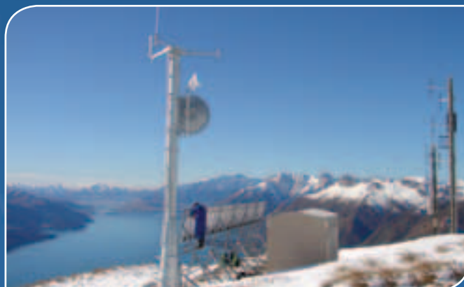
A technician installs a solar panel to the Mount Nicholas MLAT sensor at Queenstown.
