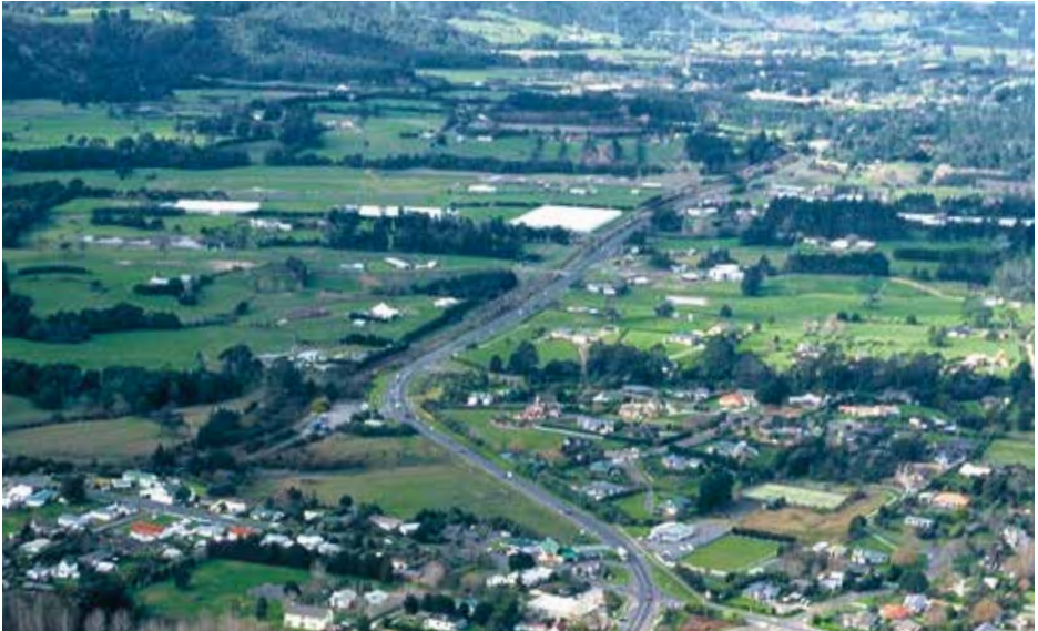
Waimauku looking northeast (The Whenuapai ATC area starts just North of Waimauku.).
