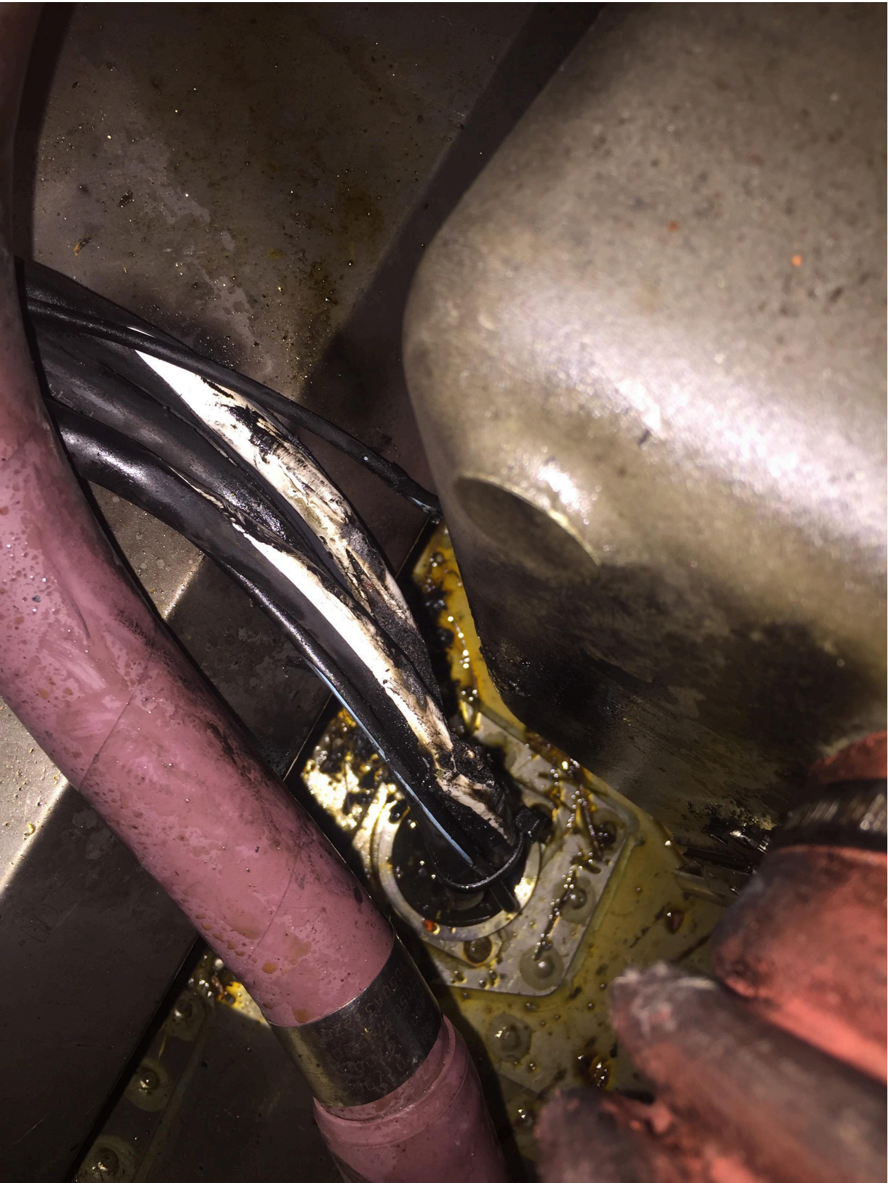
Photo 1: Plan view of the area where the generator harness is located (i.e. view from above)
